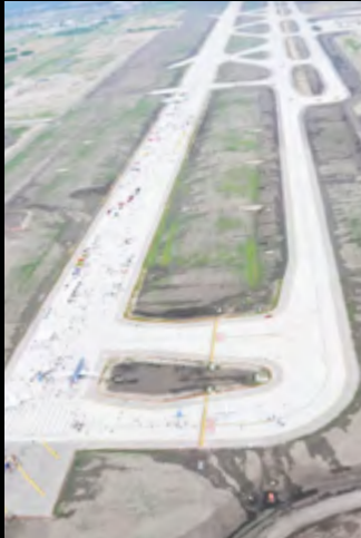
The runway, which is YYC's fourth runway, is 14,000 ft. long, 200 ft. wide and is the longest runway in Canada
